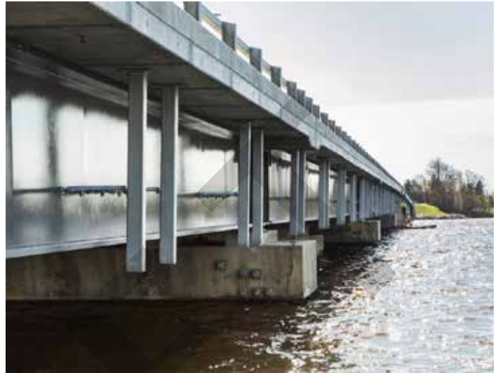
PR 313 over the Winnipeg River
